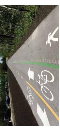
side is proposed. The pathway will provide connections A 4.5 metre off-street pathway along the entire south to existing and planned future pedestrian and cycling side of the CPT Extension and a portion of the north infrastructure, and neighbourhood destinations.
