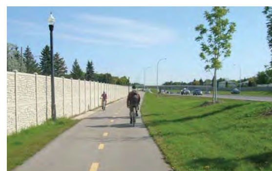
1 70m Right-of-Way for CPT locates pathway adjacent to noise attenuation wall/fencing with limited vegetative buffer
