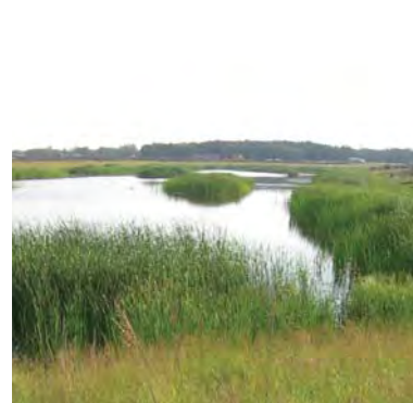
5 Naturalized storm water retention facility
