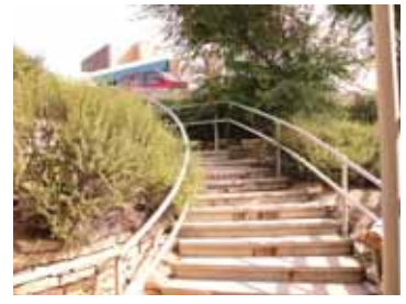
Lack of access for cyclists and wheelchair users on Portage Avenue underpass.
