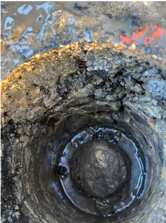
Figure 8. Photo showing Core 8 pavement showing cold mix asphalt and deteriorated concrete. Void existed between the pavement and base surface
