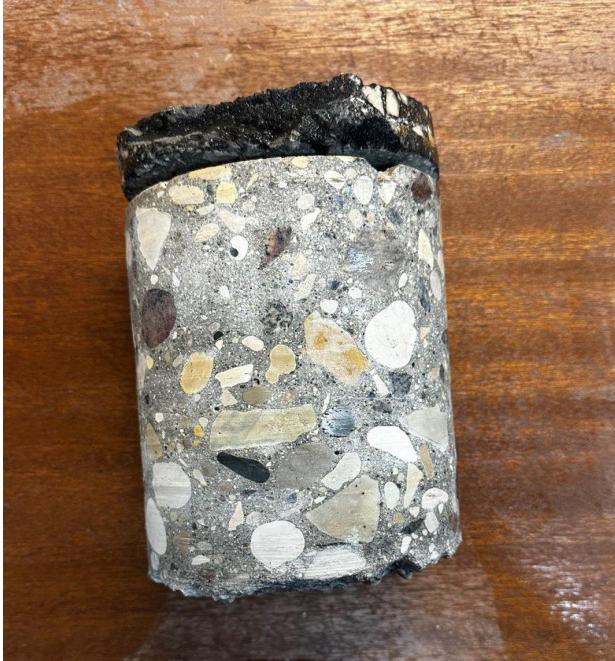
Yarwood Ave, WBL, Core 15 (Asphalt Thk 30mm; Conc Thk 200)
