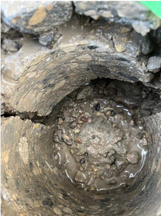
Figure 6. Photos showing Core 6 pavement showing void and deterioration of concrete at joint. Void existed between pavement and base surface
