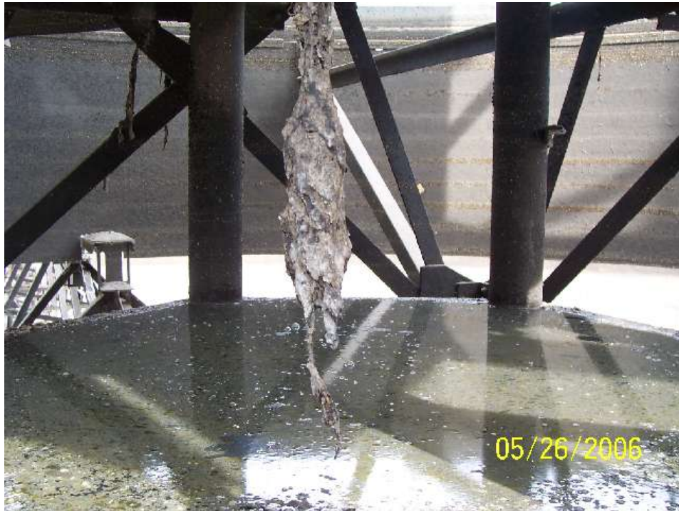
Photo 3-2 Top of Concrete Clarifier Influent Pipe/Base
