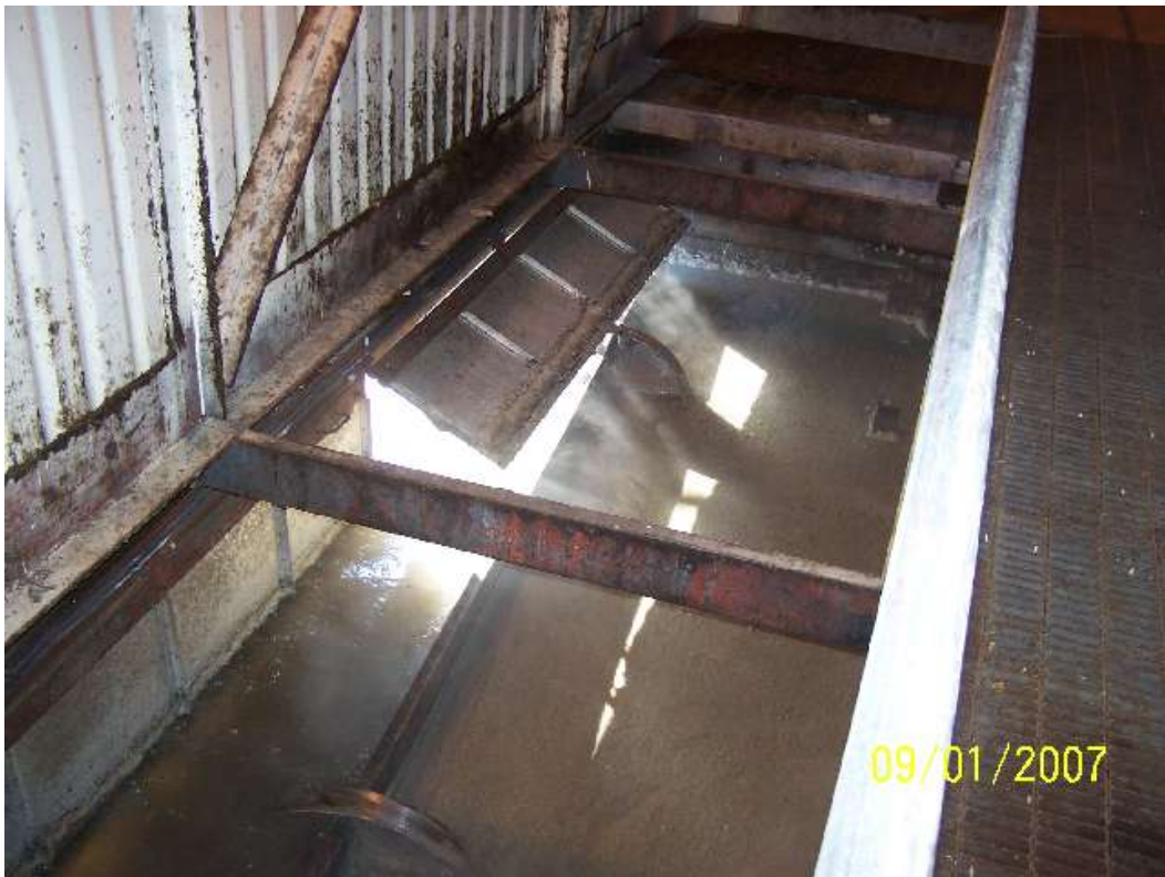
Photo 3-17 Walkway Enclosure Hinged Scum Blade Access Panels
