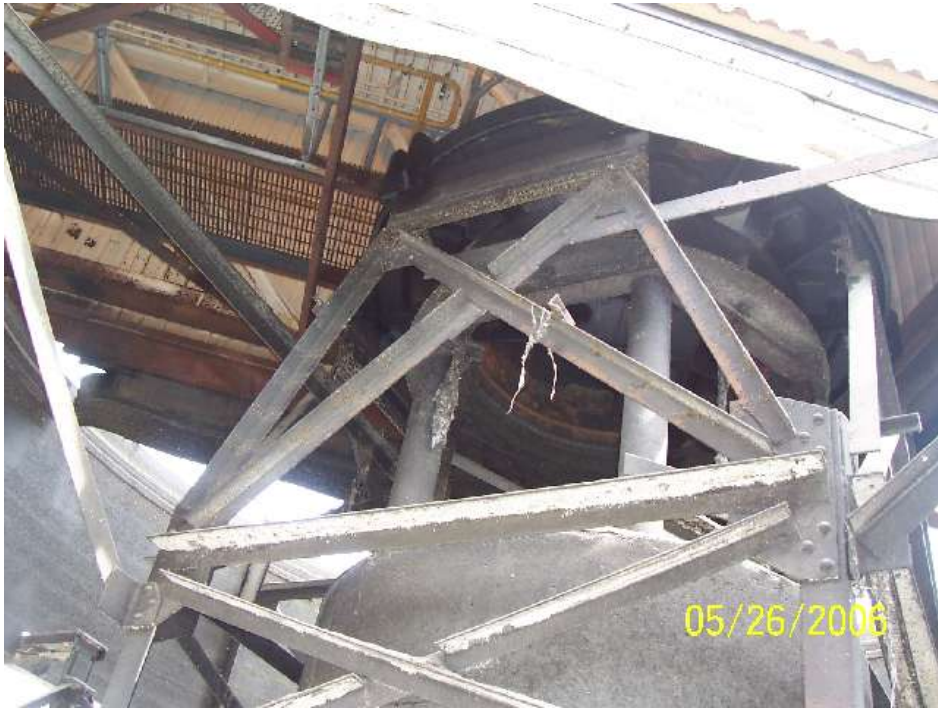
Photo 3-1 Concrete Clarifier Influent Pipe/Base
