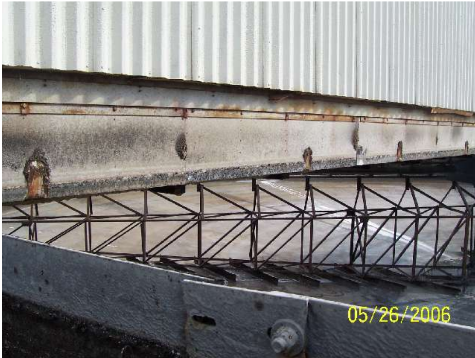
Photo 3-7 Walkway Enclosure Hinged Scum Blade Access Panels
