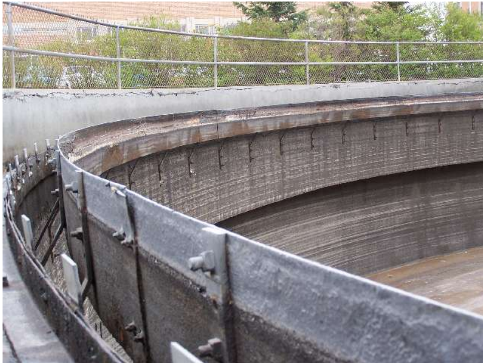
Photo 2-2 Effluent Weir & Scum Baffle
