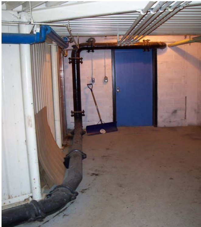
Photo 1-3B 150 mm CI Pipe-Remove
