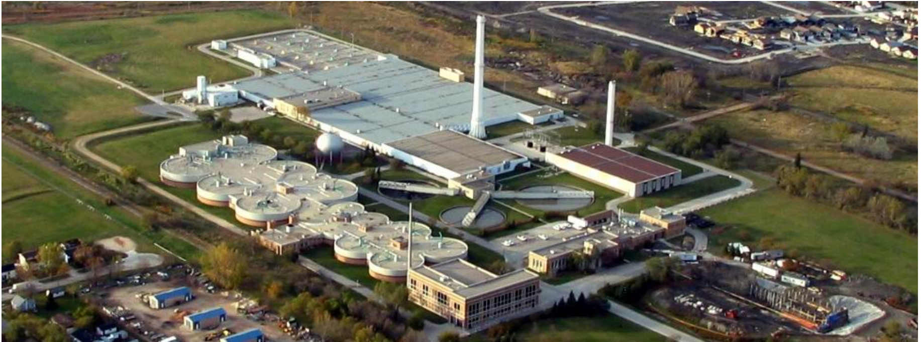
Photo 0-1 NEWPCC- Site Photo Taken in 2006
