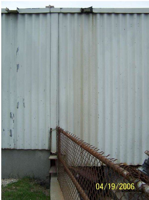
Photo 2-4 Clarifier Walkway Enclosure Connection
