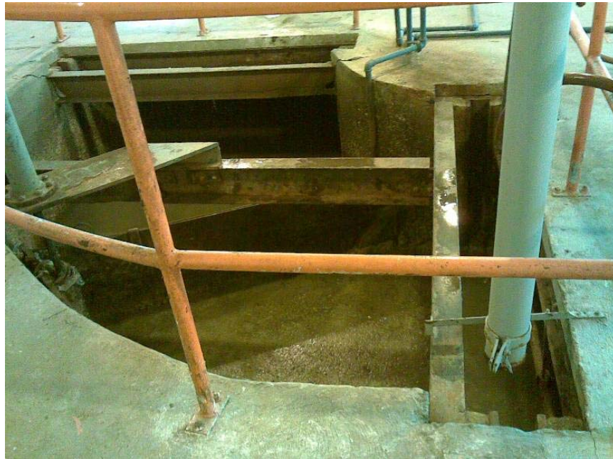
Photo 4-2 Clarifier Control Building – Center Ring – Location for Proposed Screw Conveyor
