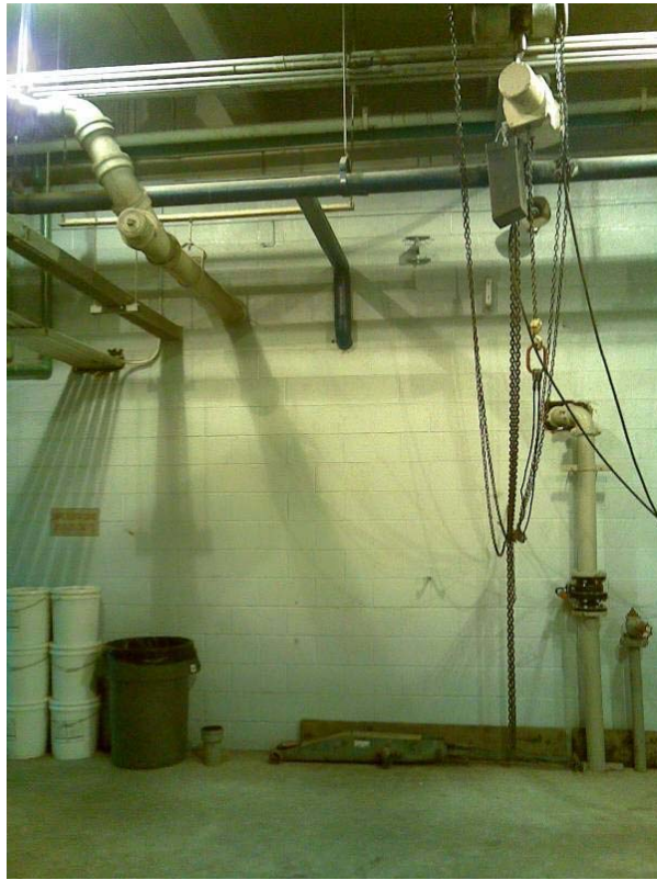
Photo 4-3 Clarifier Control Building – Location for Scum Disposal Bin
