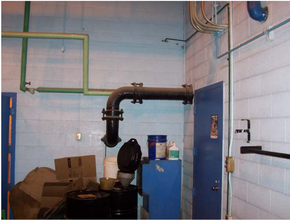
Photo 1-3C 150 mm Pipe-Removal
