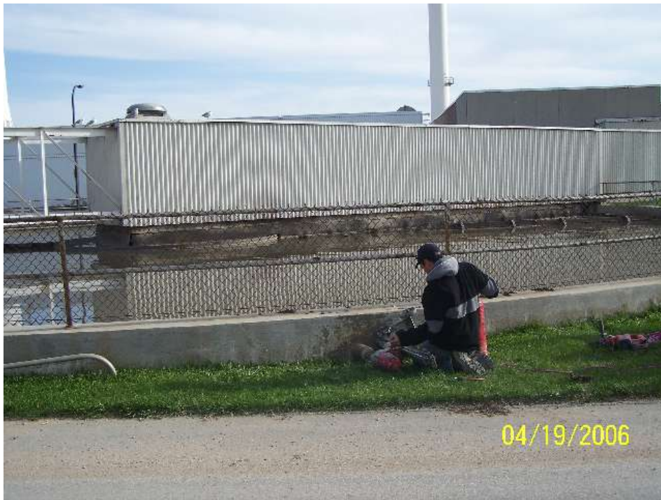
Photo 2-3 Clarifier Walkway Enclosure
