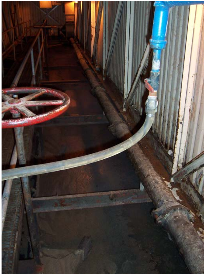
Photo 1-3A 150 mm CI Pipe-Remove
