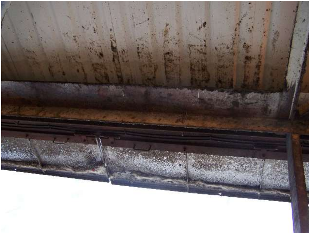
Photo 3-15 Enclosure Hinged Scum Blade Access Panels
