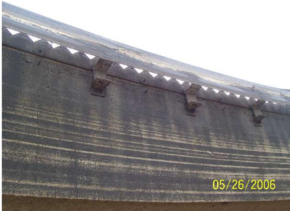
Photo 3-3 Effluent Weir & Scum Baffle
