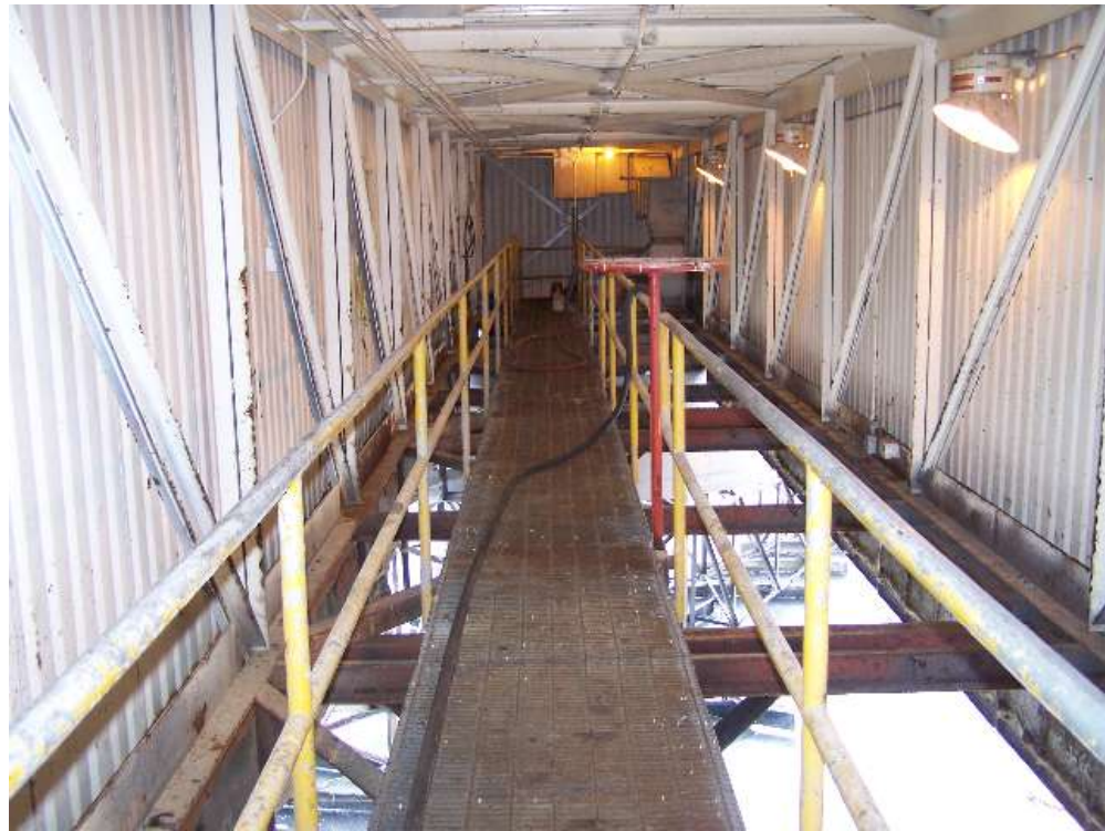
Photo 3-14 Clarifier Walkway & Enclosure
