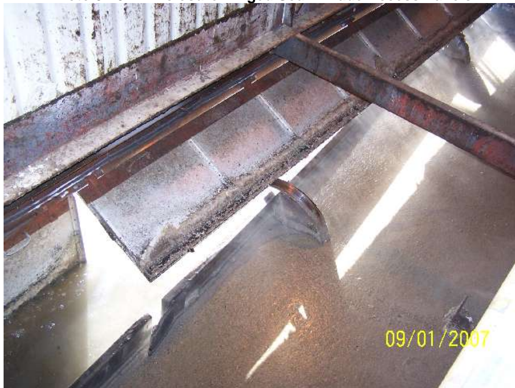
Photo 3-16 Walkway Enclosure Hinged Scum Blade Access Panels
