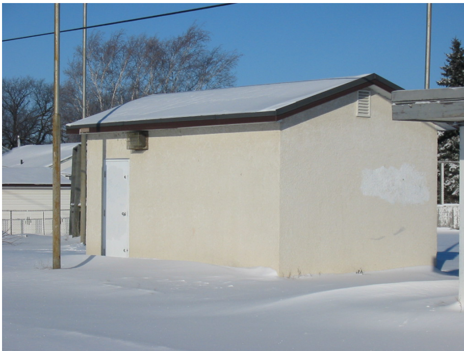
South and East side of Garage
