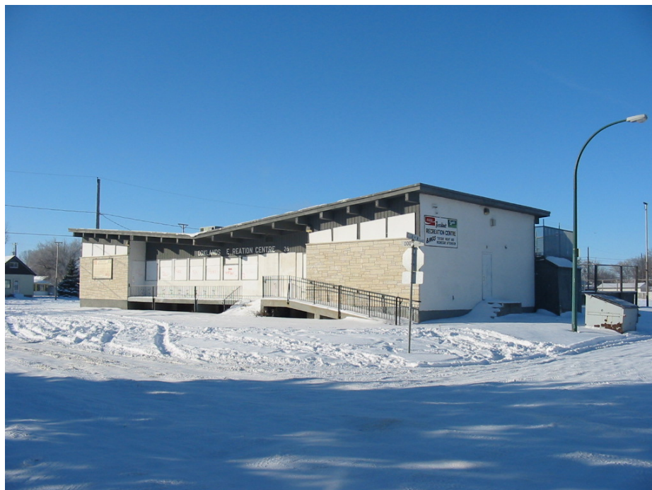
East and North side of main building
