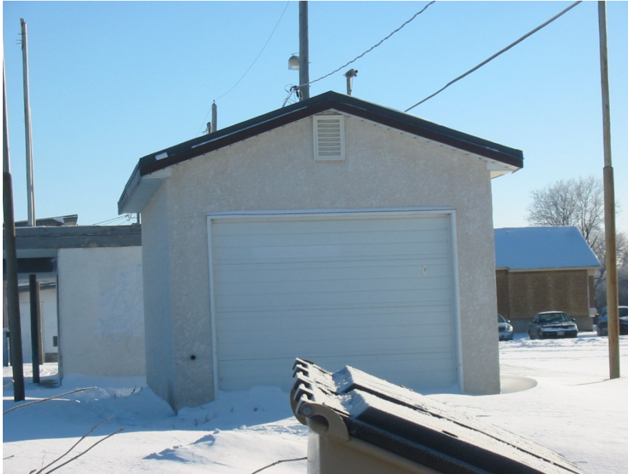
West side of Garage
