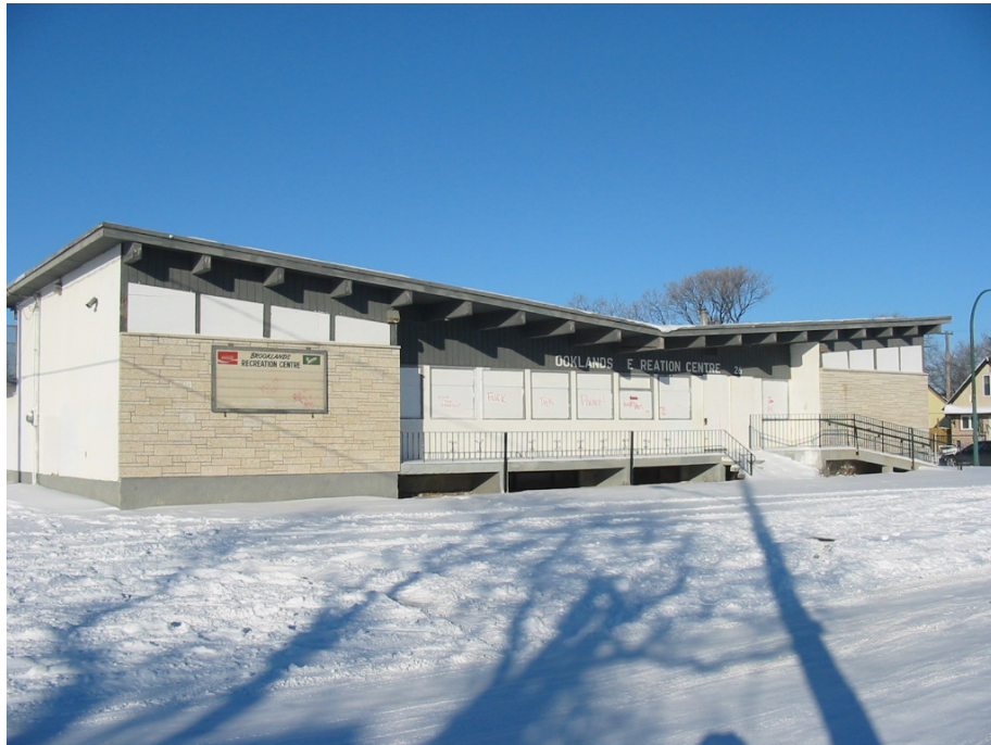
East and South side of main building
