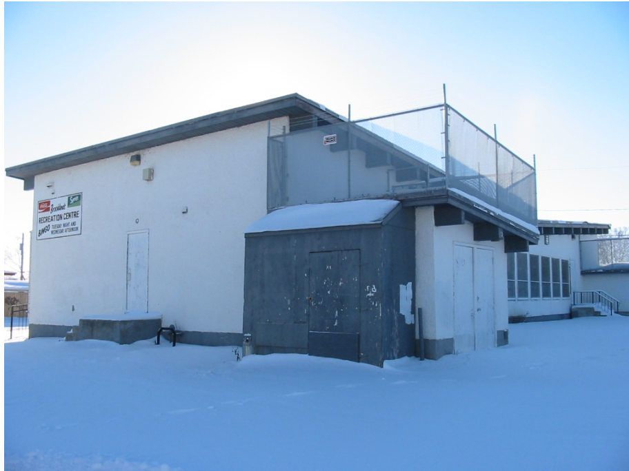
North and West side of main building
