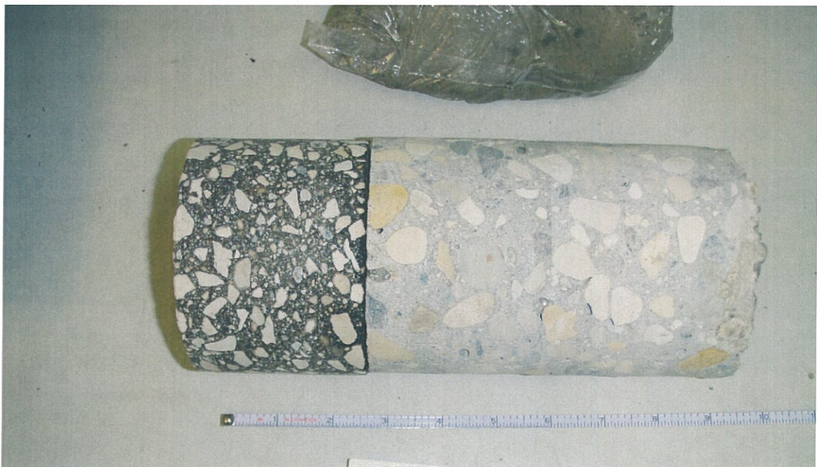
Asphalt and concrete core sample from PH-08-21
