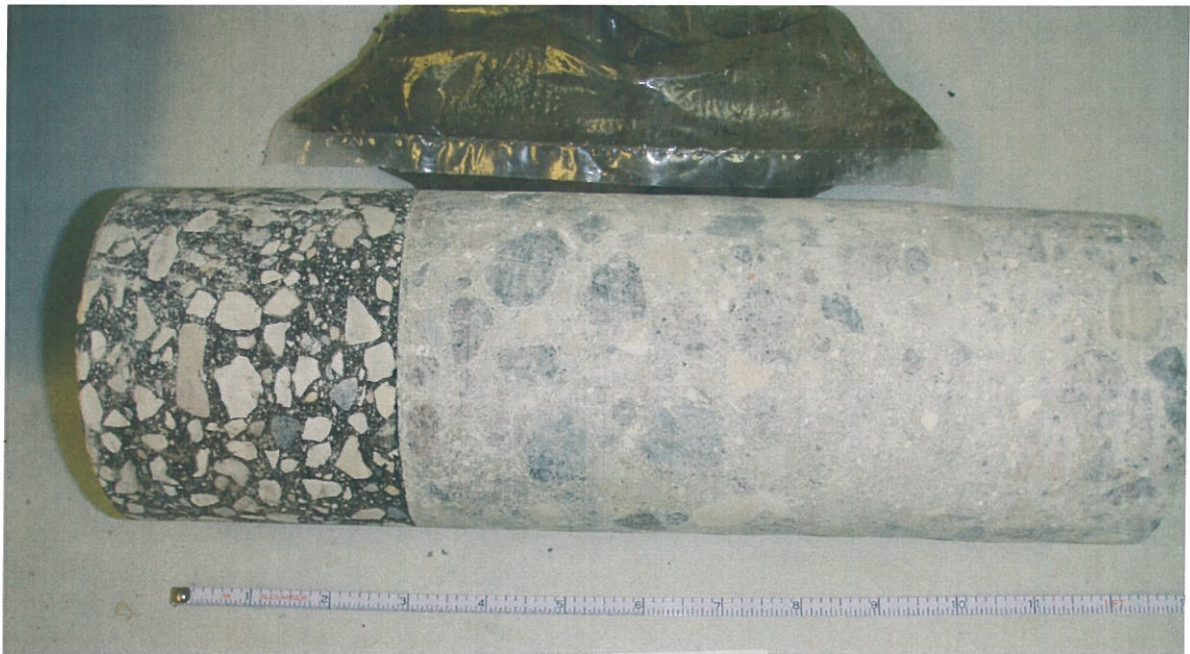
Asphalt and concrete core sample from PH-08-19
