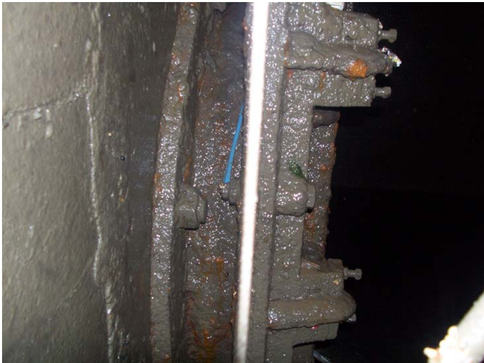
Photo 10 – Existing Slide gate to be removed
