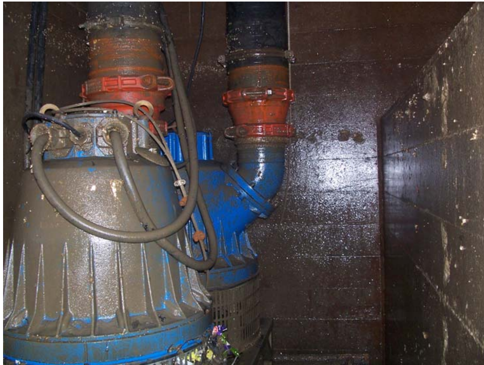
Photo 7 – Existing Pumps and Divider Walls to be Removed (Wetwell)
