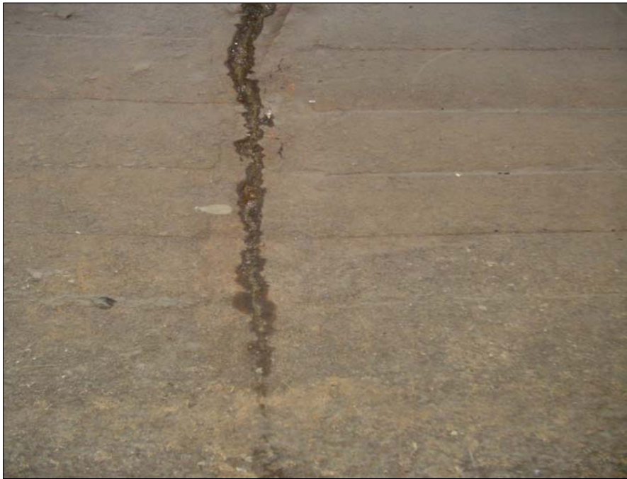
Photo 15 – Intake Pipe – Typical Wall Crack and Spalling
