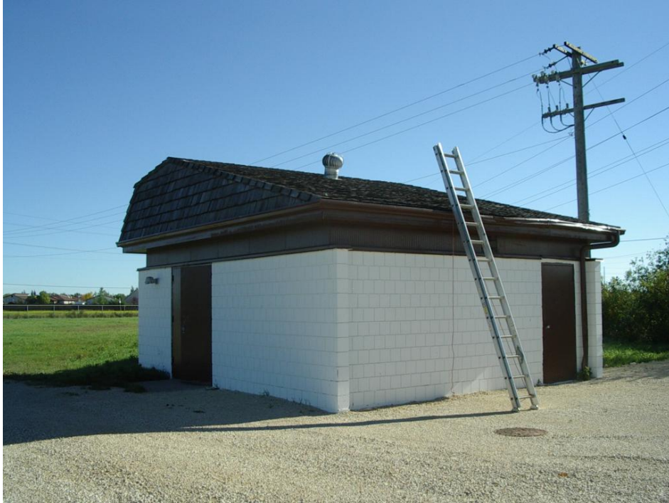
Photo 1 – Existing Building to be demolished
