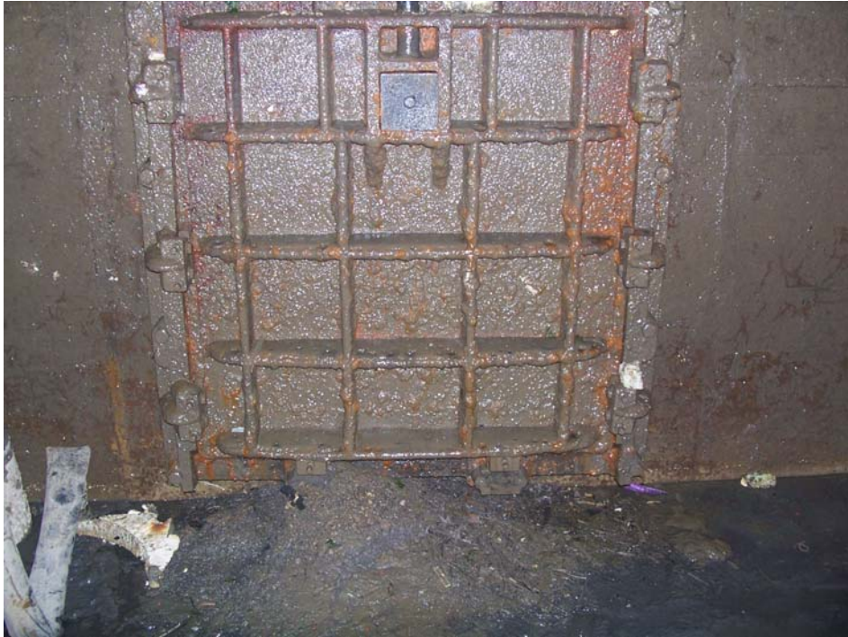
Photo 9 – Existing Slide gate to be removed
