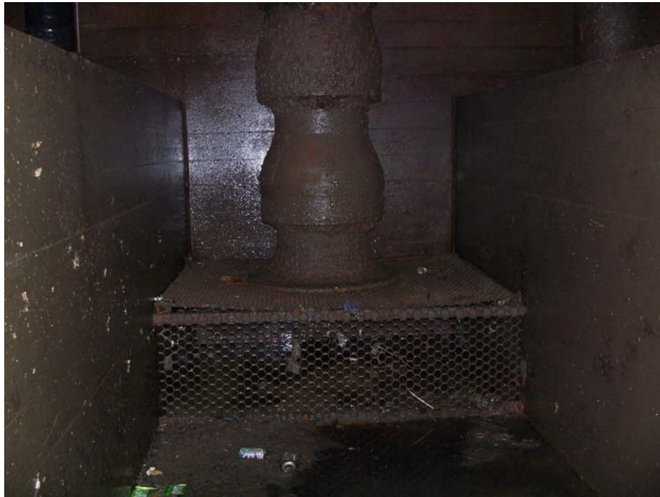
Photo 7 – Existing Pumps and Divider Walls to be Removed (Wetwell)
