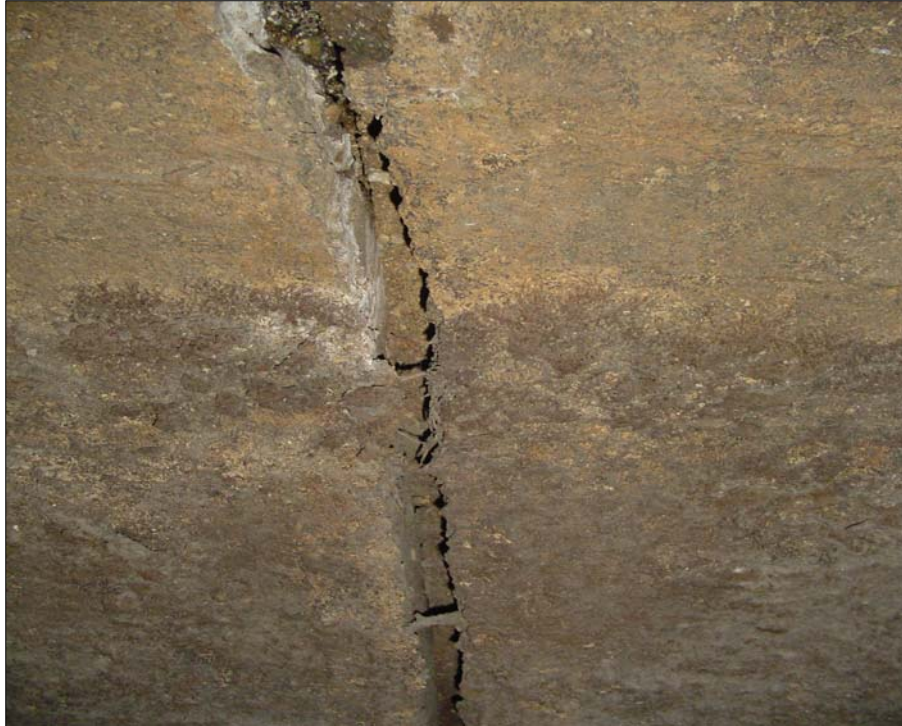
Photo 13 – Intake Pipe – Typical Wall Crack
