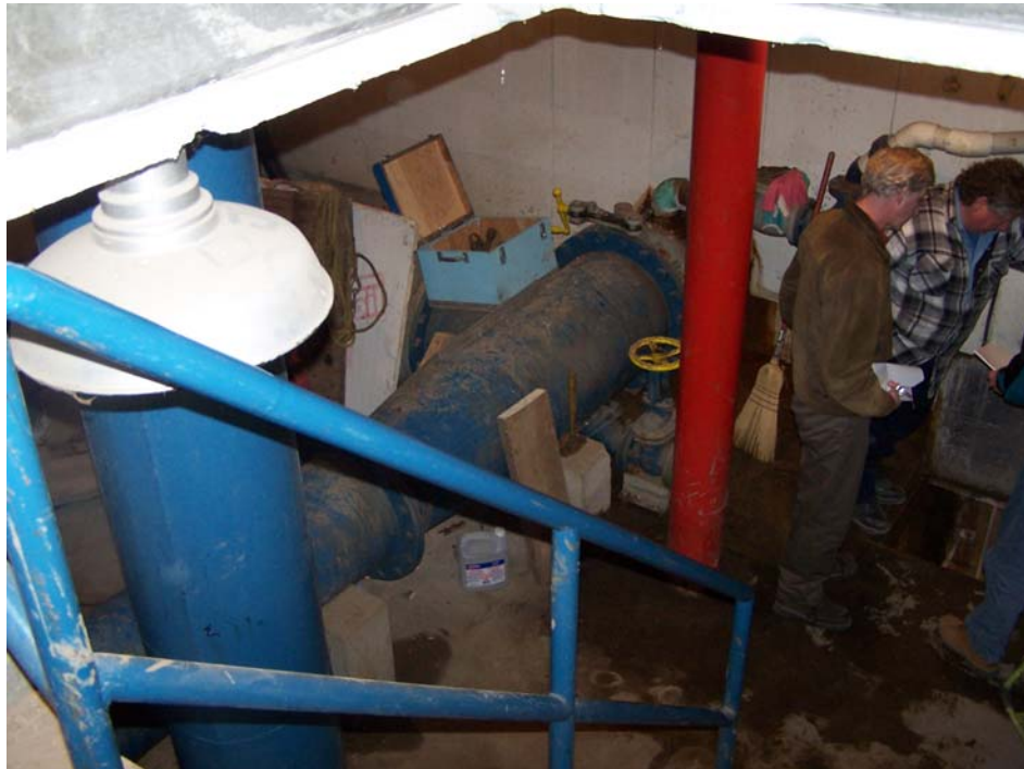
Photo 5 – Existing Piping to be removed (lower level)
