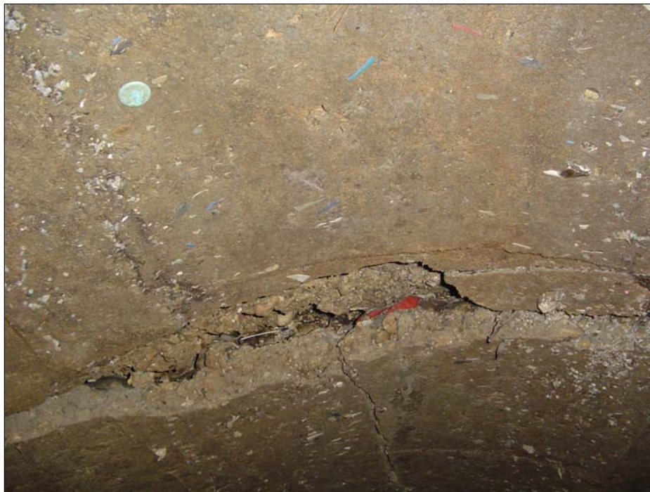
Photo 13 – Intake Pipe – Typical Wall Crack
