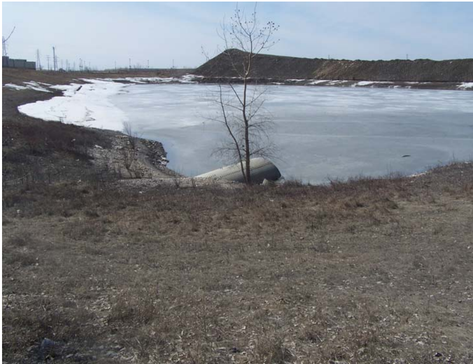
Photo 11 – Deep pond and intake pipe (April 10, 2007)
