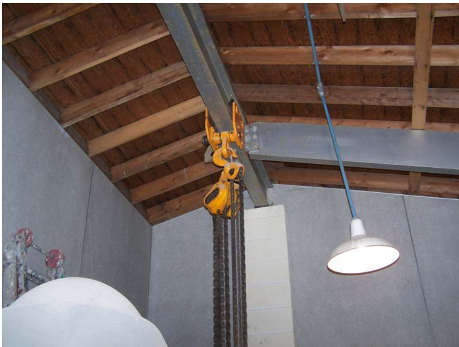
Photo 2 – Existing Asbestos wallboard to be removed (main floor).
