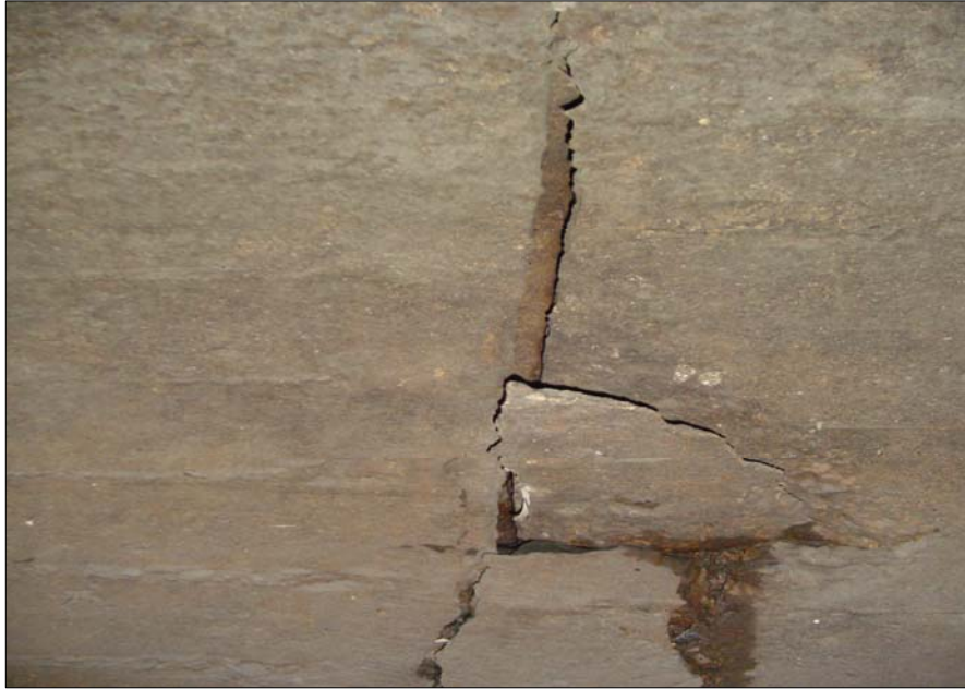
Photo 15 – Intake Pipe – Typical Wall Crack and Spalling
