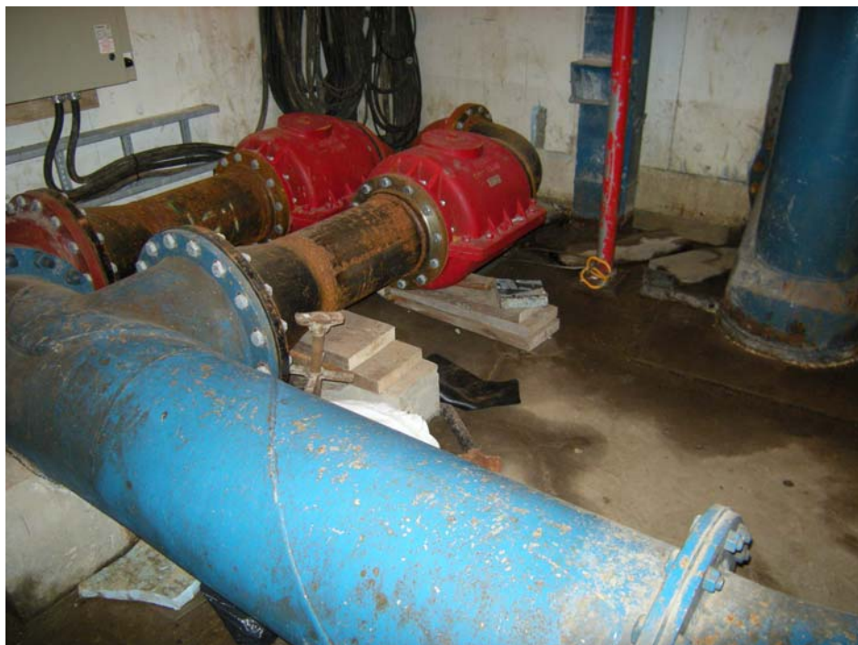
Photo 6 – Existing Piping to be removed (lower level)
