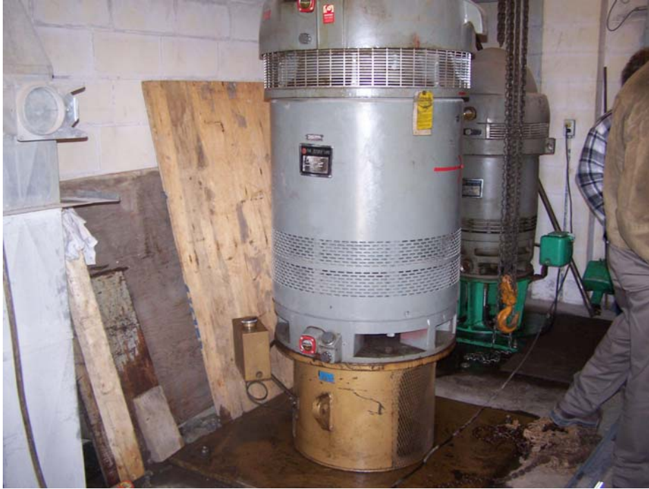
Photo 3 – Existing Electrical to be removed (main floor)
