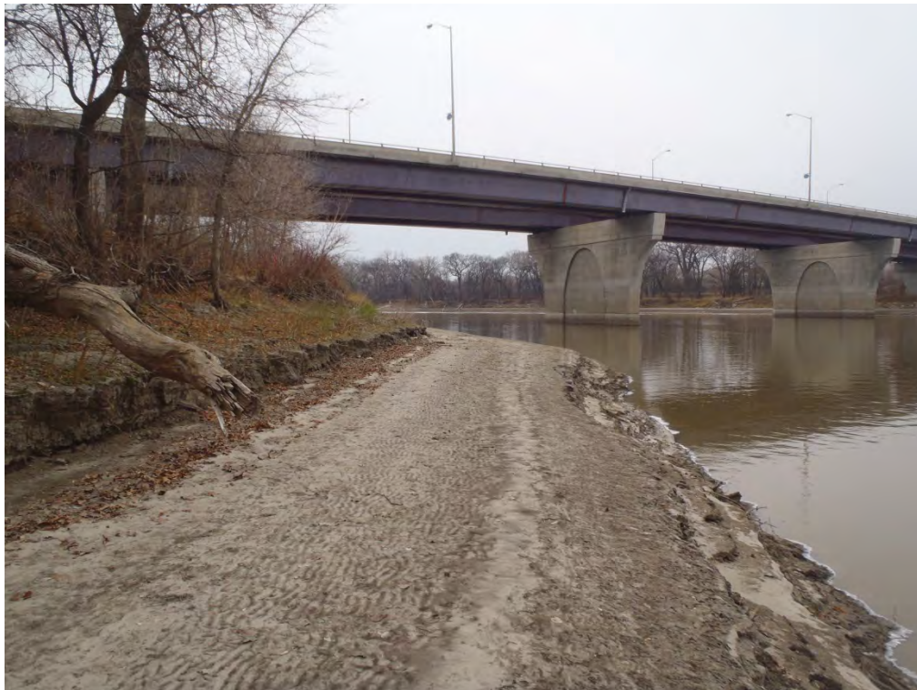
Figure 05: East Riverbank (November 8, 2013)
