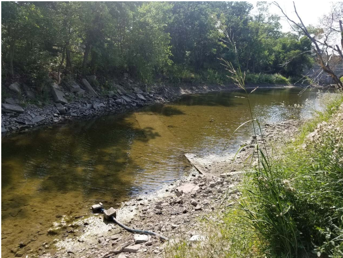
Figure 4 – Concrete Encasement Visible on Creek Bottom.
