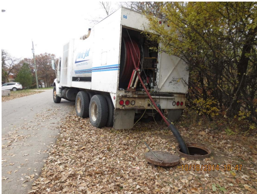
Figure 6 – Existing Chamber Access Location on South Side of Sturgeon Creek.
