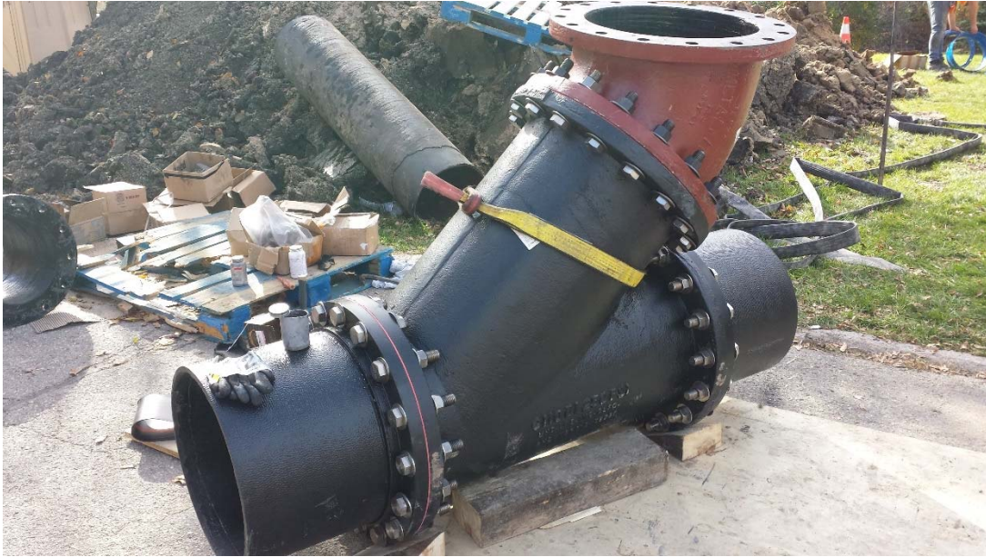
Figure 1 – Tool Launch Wye with Temporary 45 Degree Bend.
