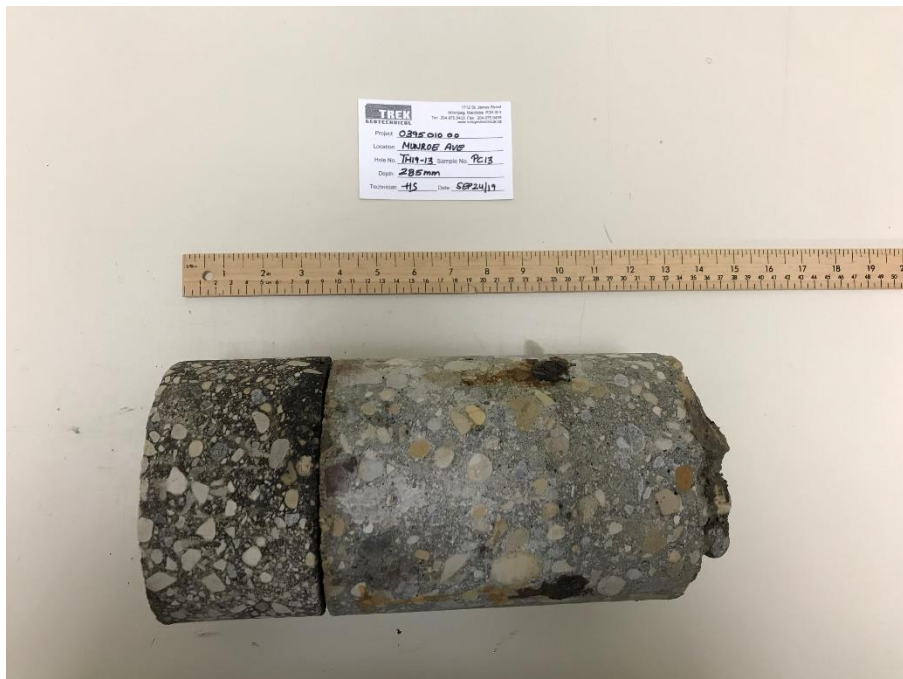
Photo 13: Pavement Core Sample at Test Hole TH19-13
