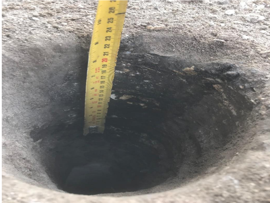
Photo 23: Pavement Core Measurement at Test Hole TH19-23
