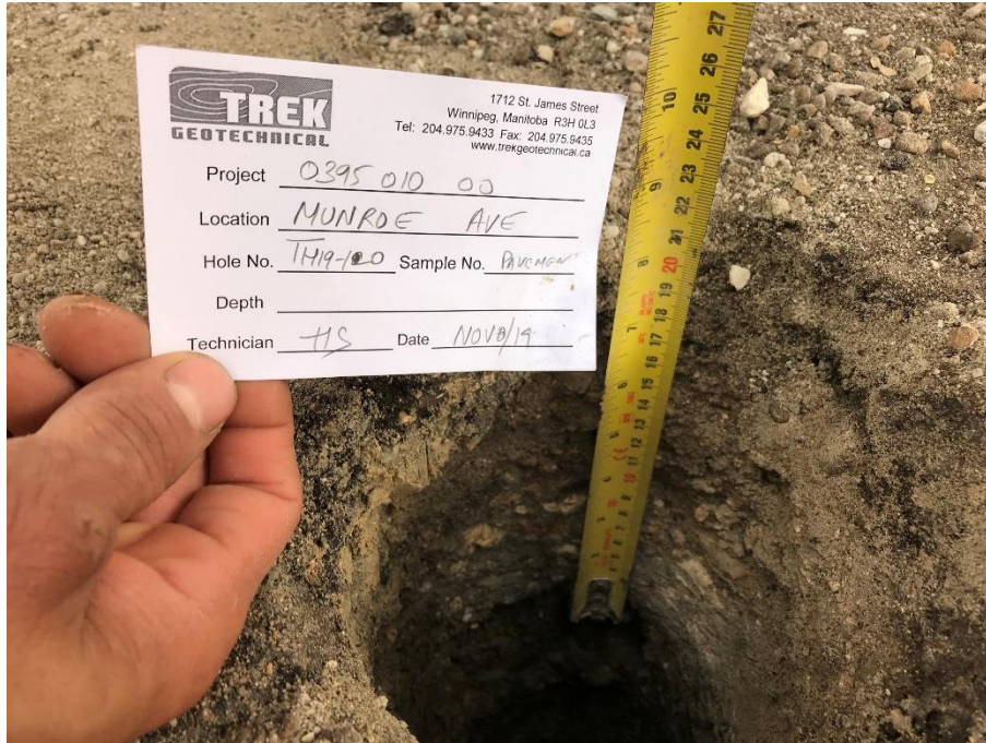
Photo 10: Pavement Core Measurement at Test Hole TH19-10
