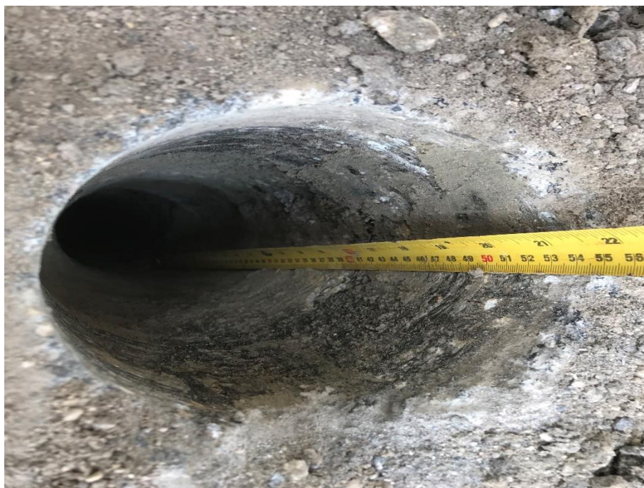
Photo 24: Pavement Core Measurement at Test Hole TH19-24
