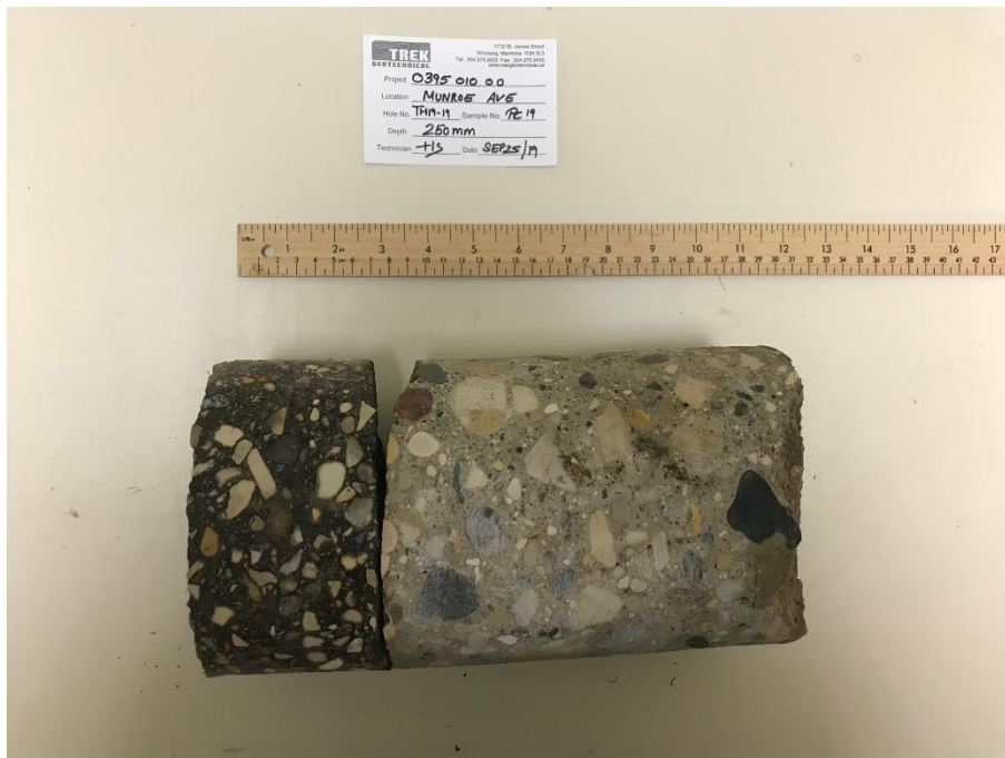
Photo 19: Pavement Core Sample at Test Hole TH19-19
