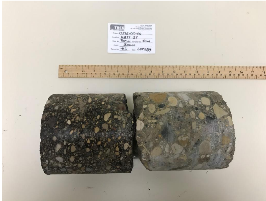
Photo 1: Pavement Core Sample at Test Hole TH19-01
