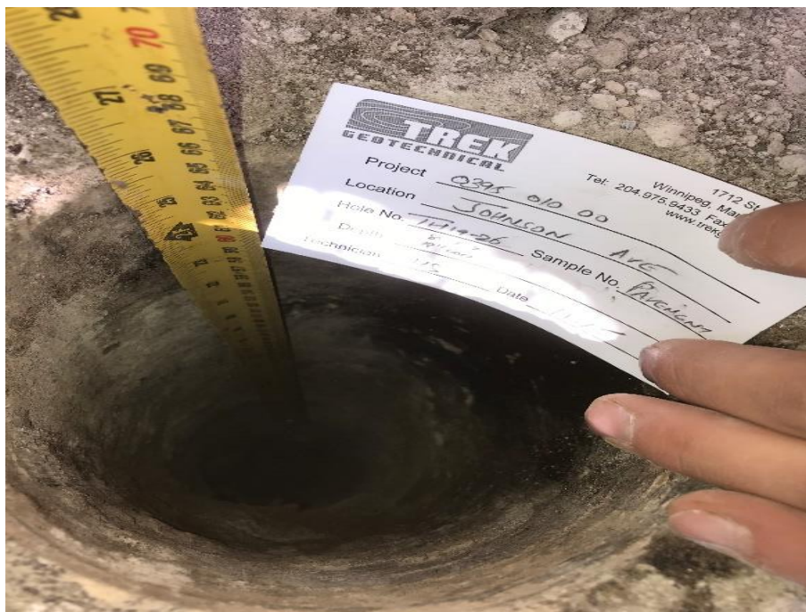
Photo 26: Pavement Core Measurement at Test Hole TH19-26
