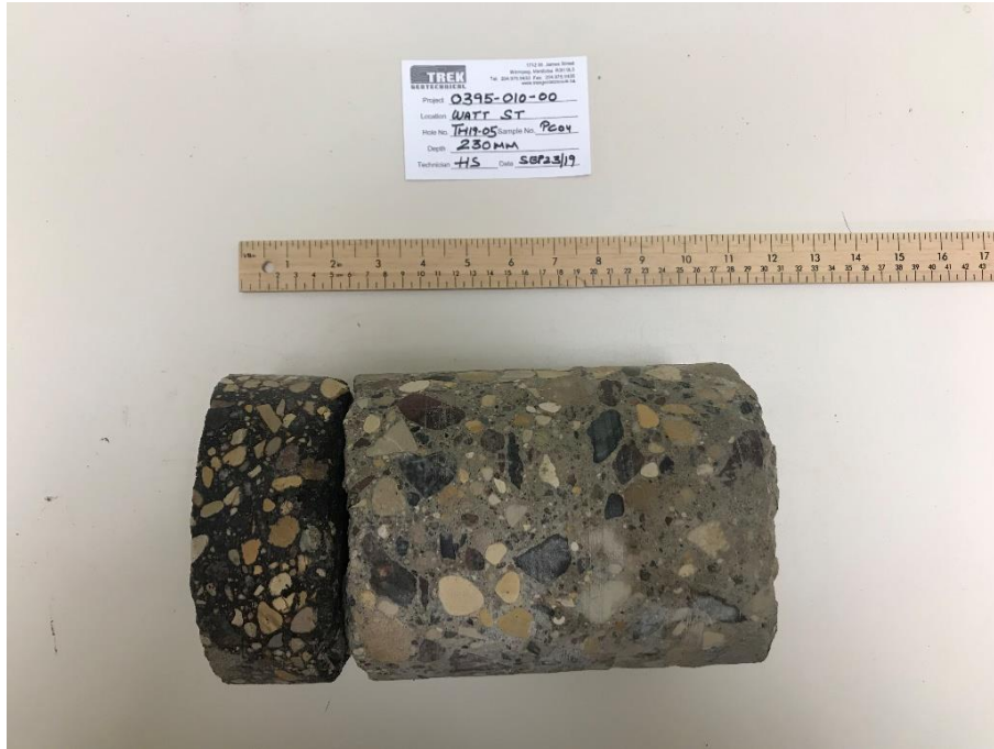
Photo 5: Pavement Core Sample at Test Hole TH19-05
