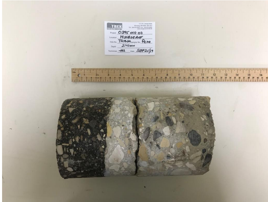
Photo 20: Pavement Core Sample at Test Hole TH19-20
