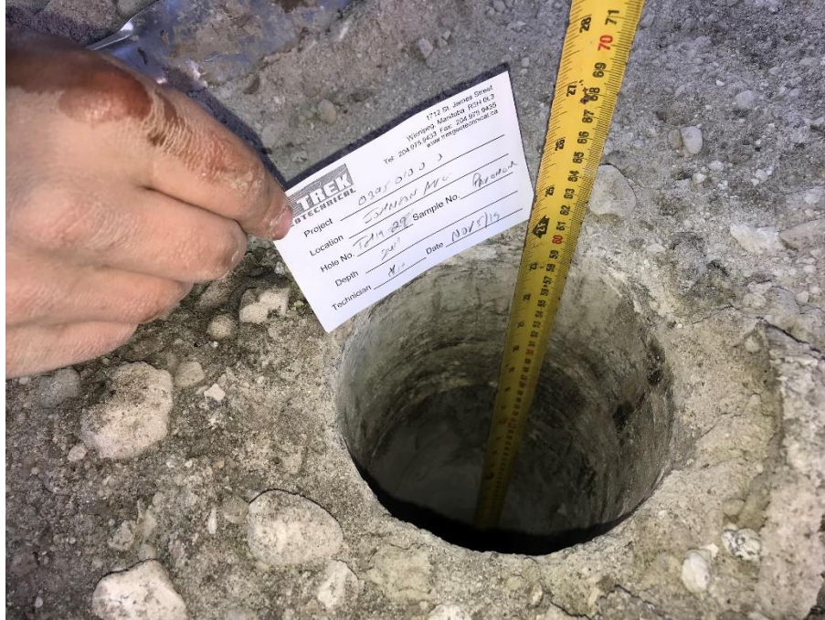
Photo 29: Pavement Core Measurement at Test Hole TH19-29
