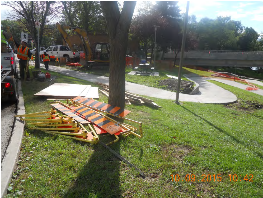
Figure 10 – General Site Layout on North Side of Crossing, looking East.
