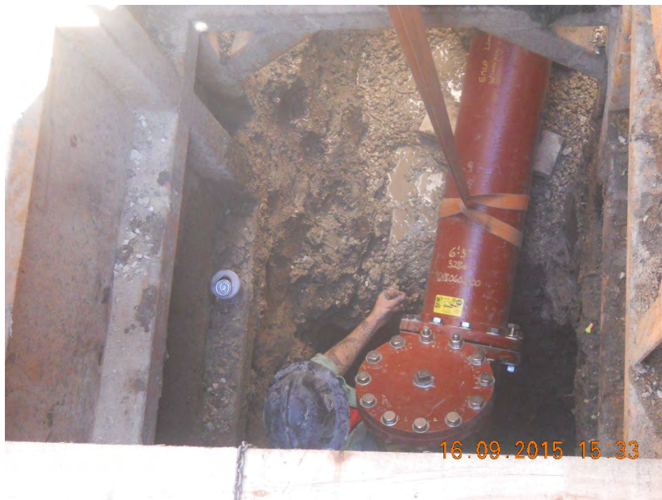
Figure 2 – Existing Launch Wye Installed on North Side of River.
