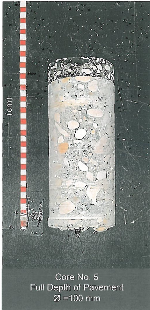
Photograph 5: Intact specimens from Keewatin Street
