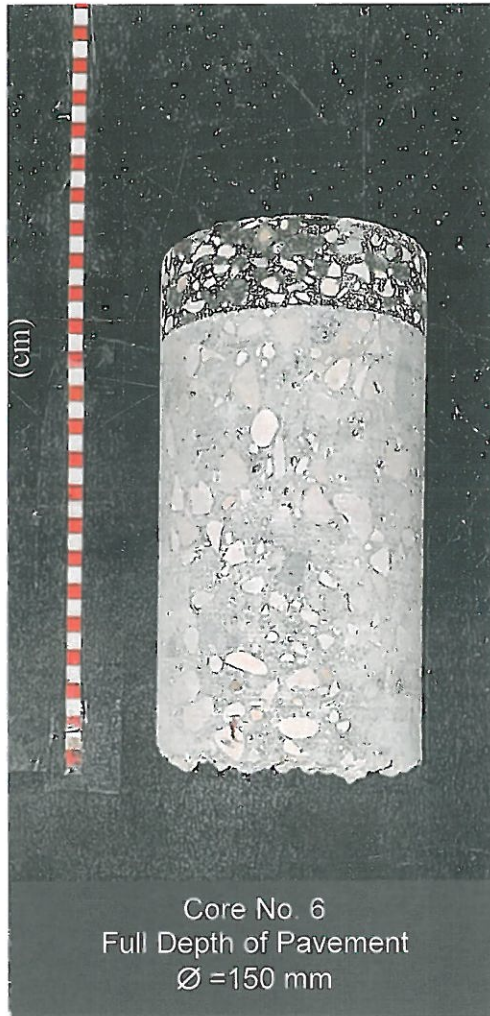
Photograph 6: Intact specimens from Keewatin Street
