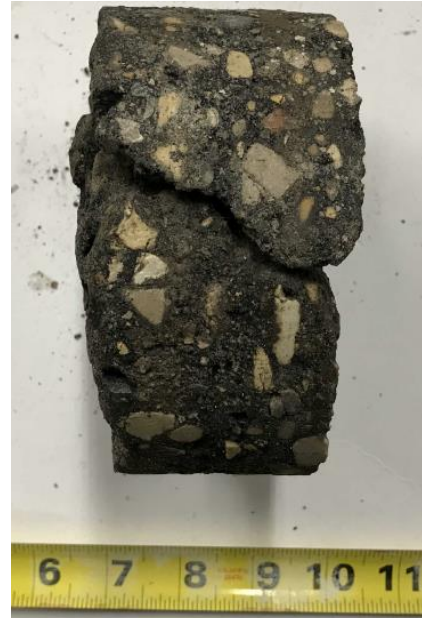
DAY-02: Asphalt Layer, Profile View
