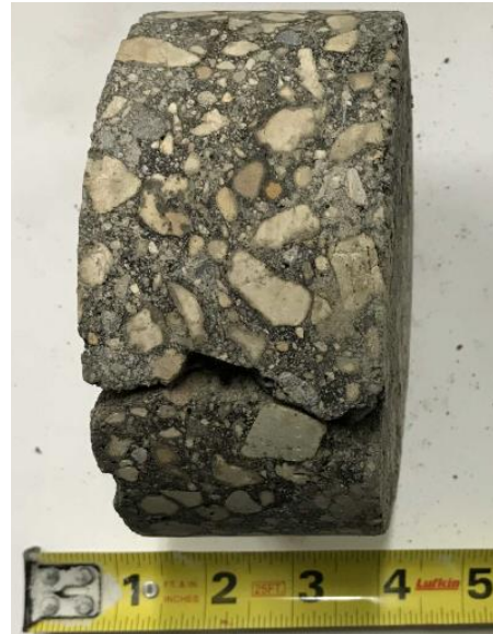
DAY-01: Asphalt Layer, Profile View
