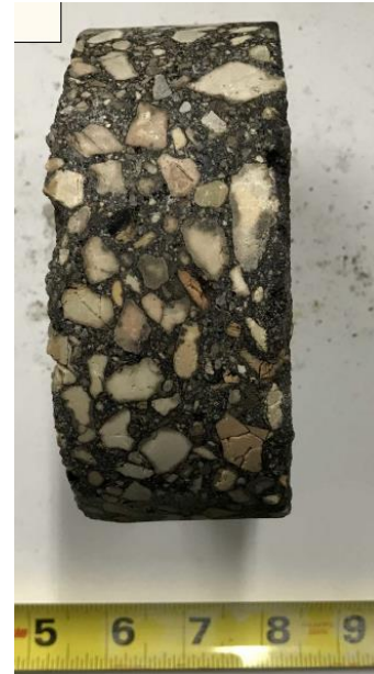
DAY-04: Asphalt Layer, Profile View
