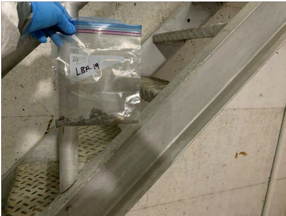
Photo 33: General view of the paint chip sample LBP-19 location on the access stairs in the motor room. (April 27, 2021)
