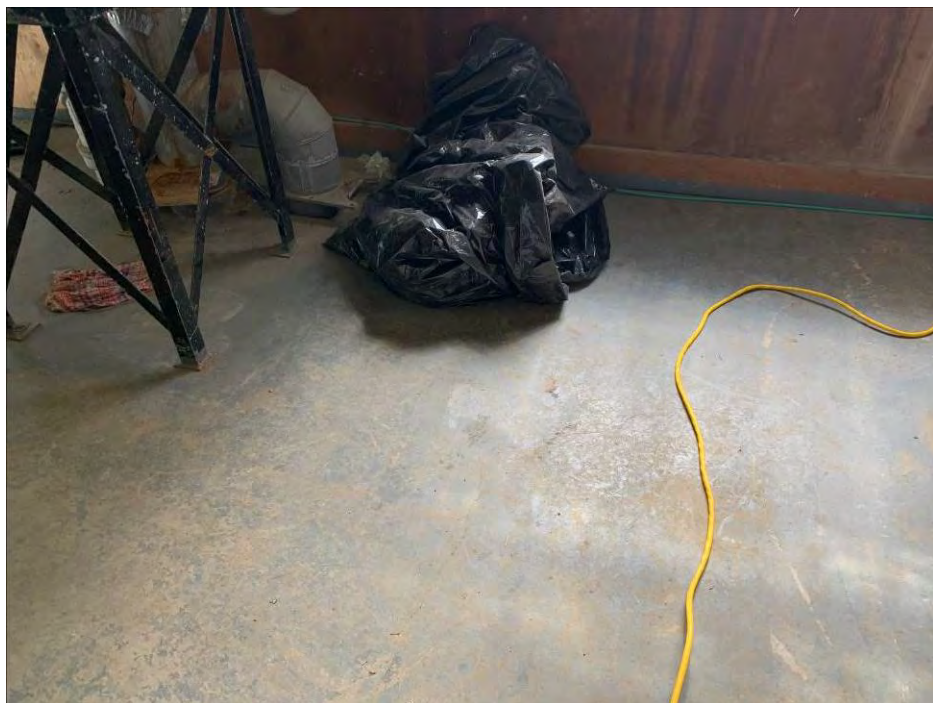
Photo 20: General view of the flooring of the main floor. (April 27, 2021)
