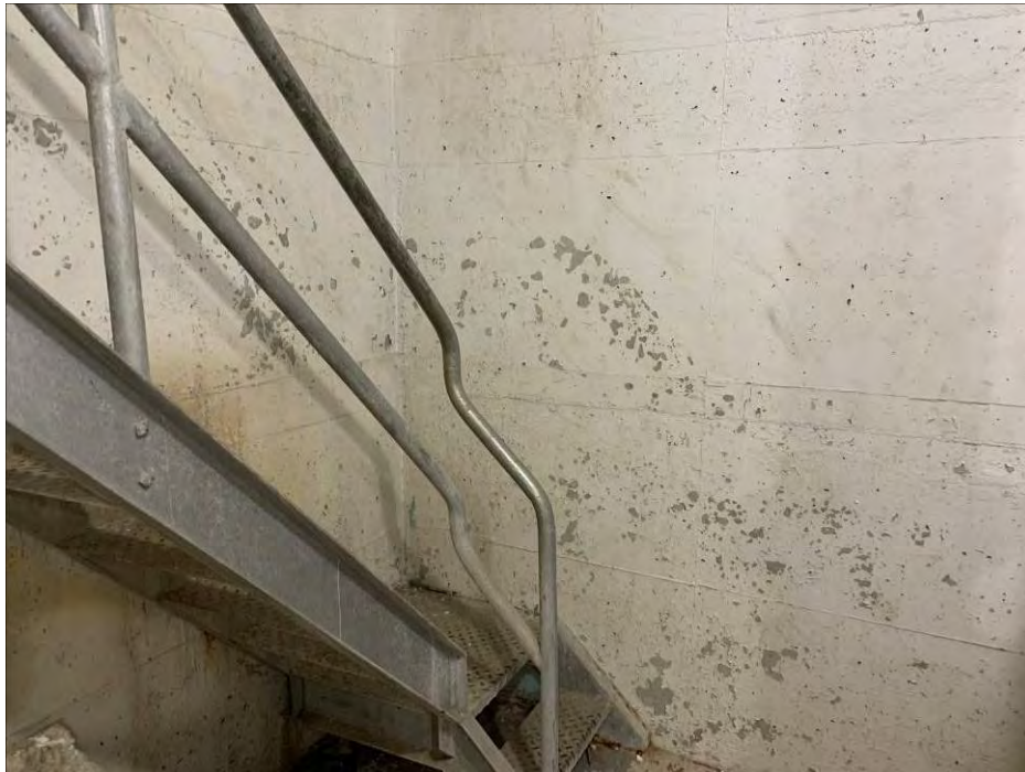
Photo 28: General view of the painted walls in the pump chamber. (March 15, 2018)
