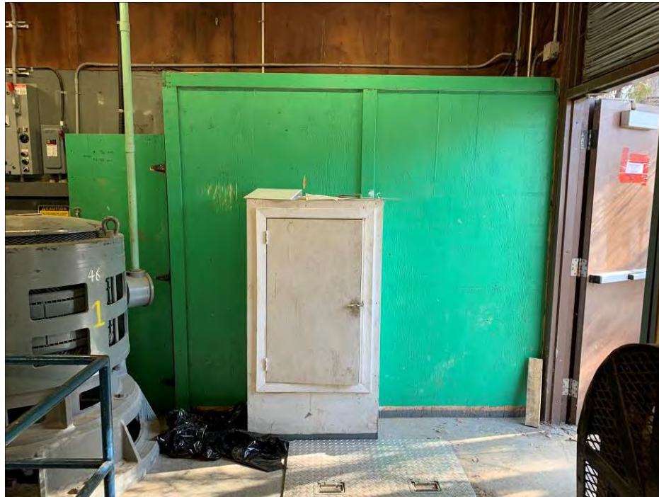
Photo 7: General view of the vestibule for the access stairs and an attached cupboard on the north wall of the main floor. (April 27, 2021)
