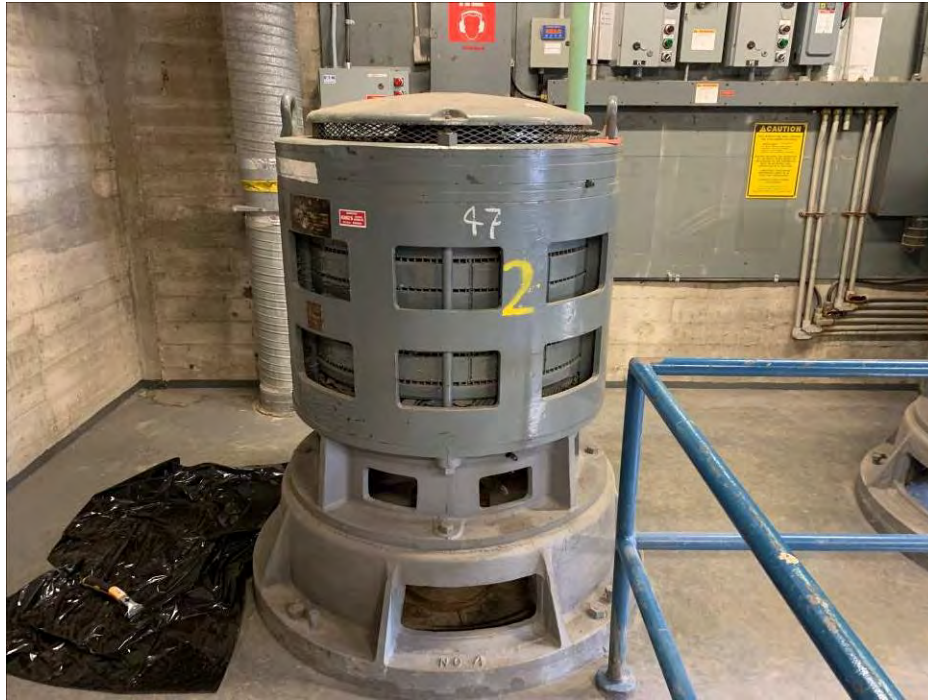
Photo 3: General view of the top drive unit for the centrifugal pump P-47. (April 27, 2021)
