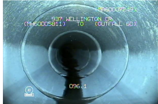
Photo 2: Approx. Sta. 1+96.1 looking d/s
