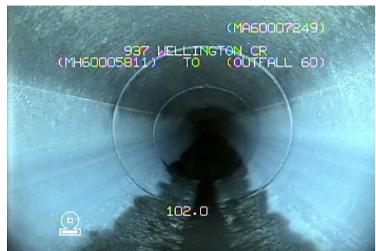
Photo 6: Approx. Sta. 2+02 looking d/s
