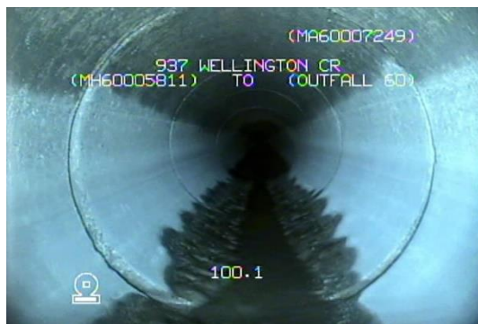
Photo 5: Approx. Sta. 2+00.1 looking d/s
