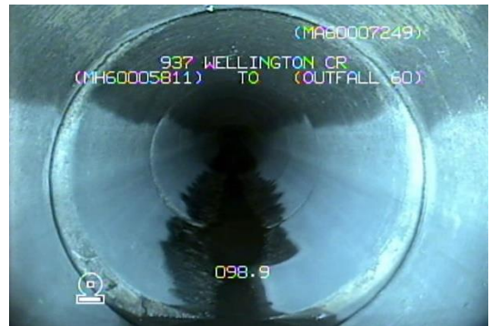
Photo 4: Approx. Sta. 1+98.9 looking d/s
