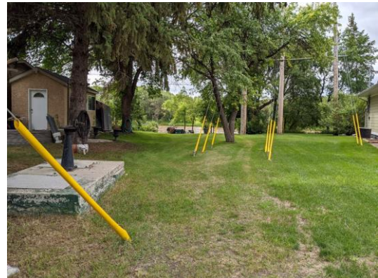
Photo 4: 2464 Assiniboine Crescent – Looking south from existing chamber
