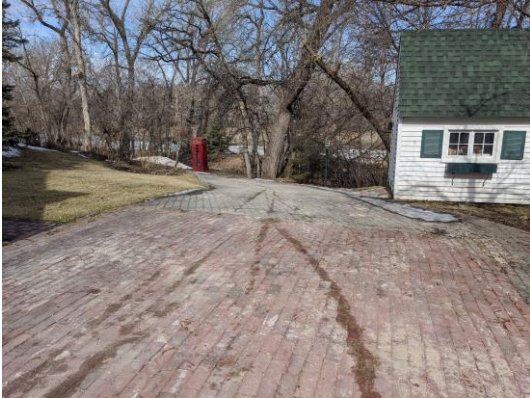
Photo 7: Wellington Crescent – Looking northwest at back of 925 Wellington Cr. property
