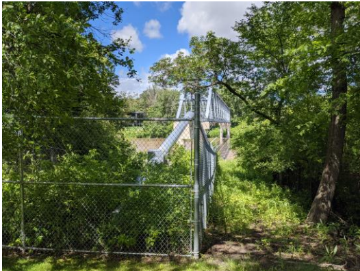
Photo 3: Wellington Crescent – Looking north at existing feedermain overhead crossing
