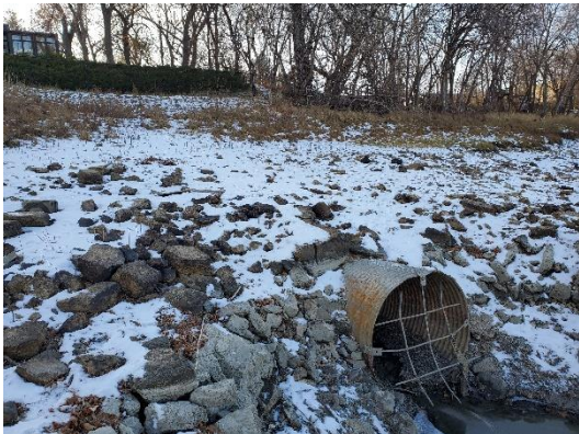
Photo 3: 300 Dunkirk Drive – Looking south at pipe outlet
