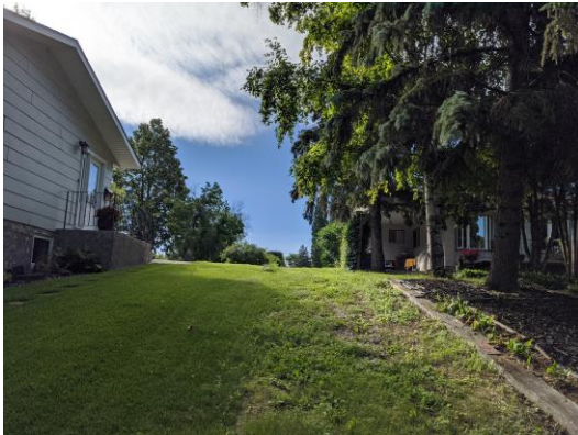
Photo 3: 50 Eastwood Drive – Looking southeast along pipe alignment between 34 Eastwood Dr. and 50 Eastwood Dr.
