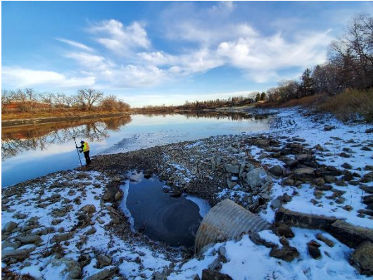
Photo 1: 300 Dunkirk Drive – Looking north at pipe outlet/shoreline
