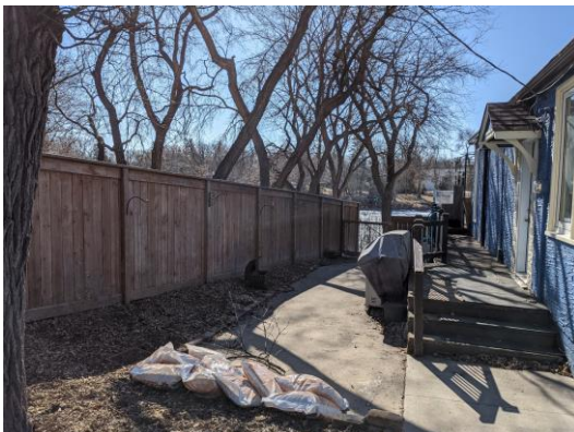
Photo 5: 2782 Assiniboine Avenue – Looking south at intermediate manhole location (manhole is along fenceline)
