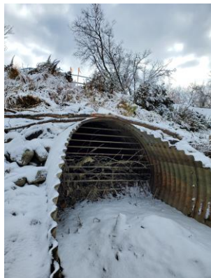
Photo 5: 1 Hart Avenue – Looking south at pipe outlet
