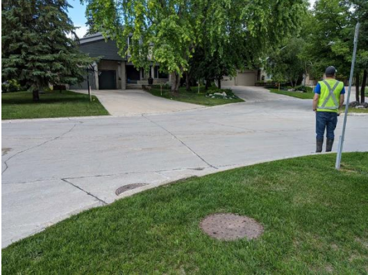
Photo 1: 3087 Vialoux Drive – Looking north along pipe alignment towards 3087 Vialoux Dr.
