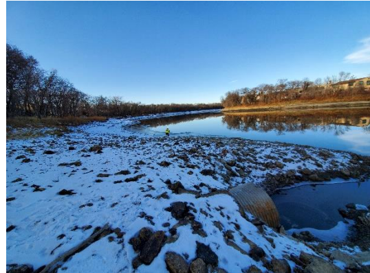
Photo 2: 300 Dunkirk Drive – Looking southwest at pipe outlet/shoreline
