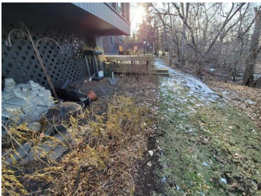
Photo 5: 300 Dunkirk Drive – Looking southeast along pipe alignment
