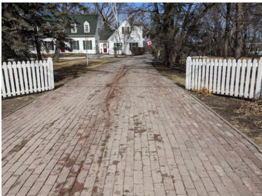
Photo 5: Wellington Crescent – Looking north along 925 Wellington Cr. driveway
