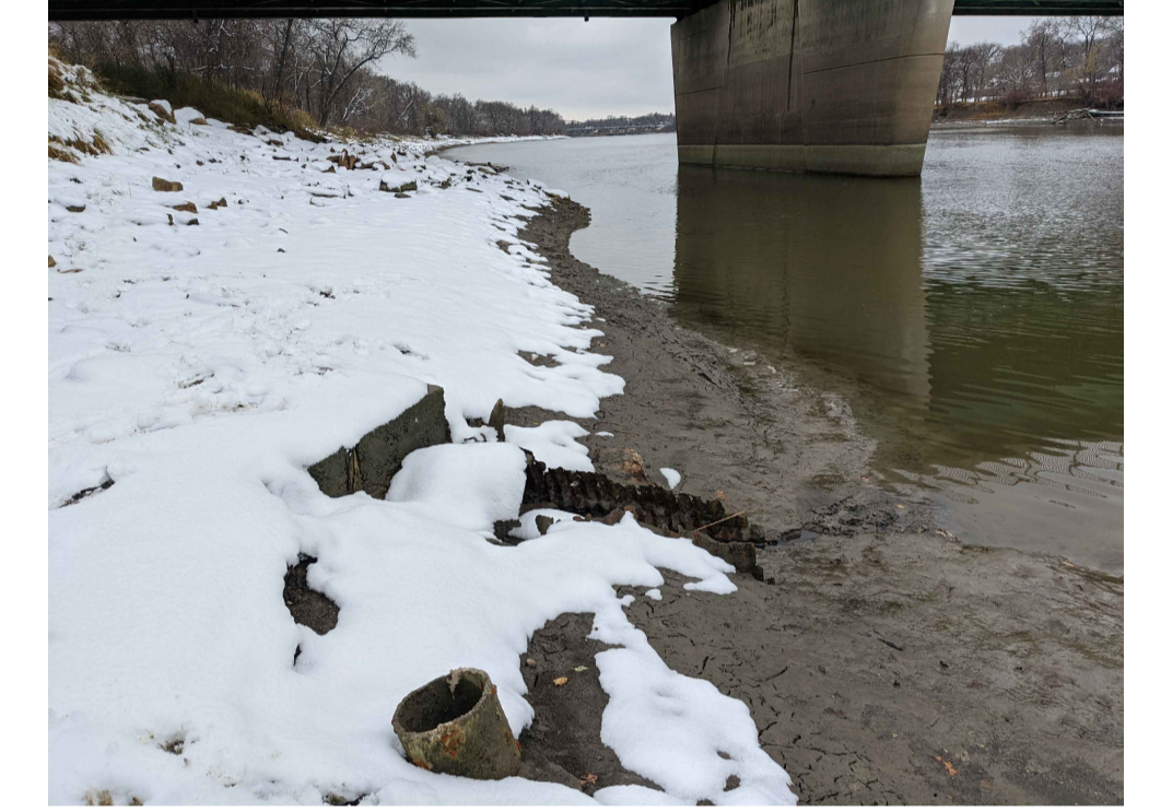
PIPE OUTLET LOOKING WEST DATE 2020-10
