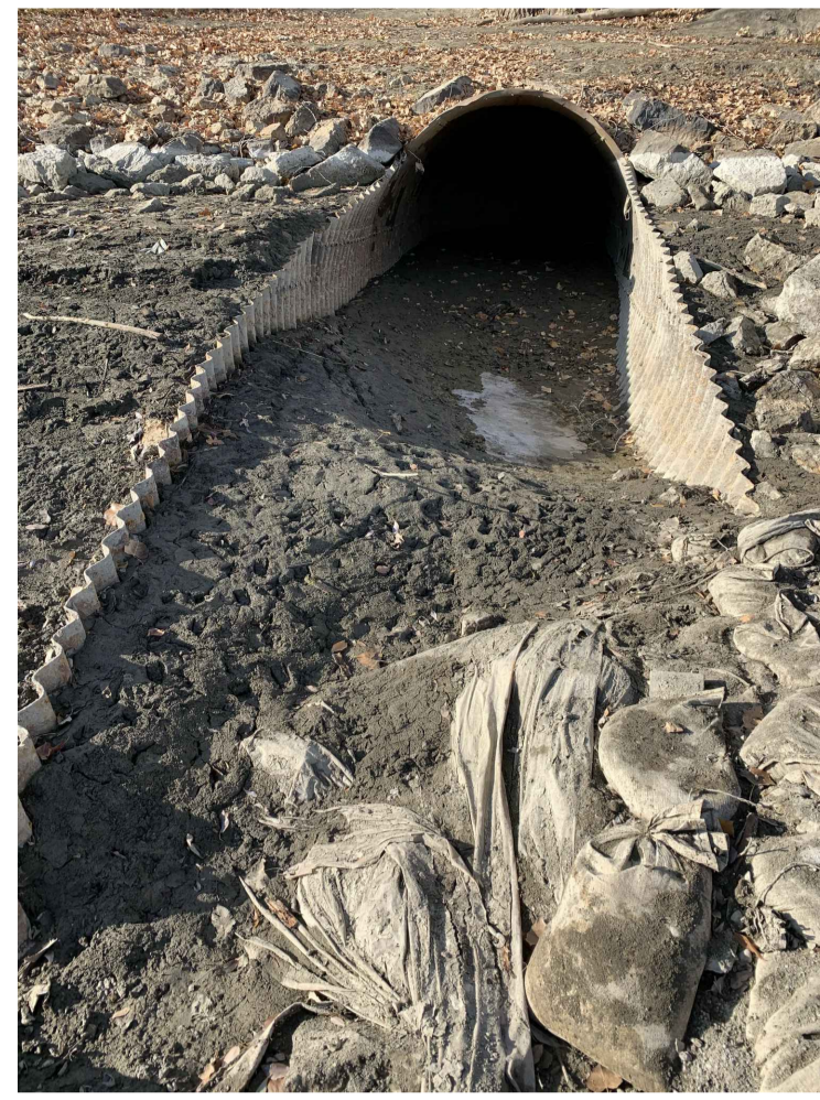
PIPE OUTLET DATE 2020-11
