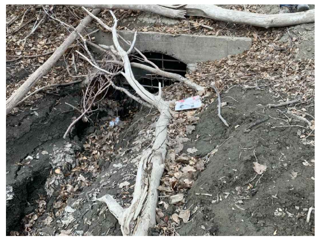
PIPE OUTLET DATE 2021-03
