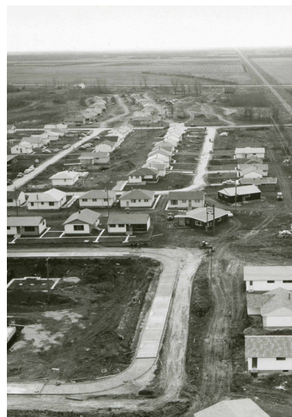
Houses under construction in Windsor Park, circa 1956. Photo by David Portigal.
