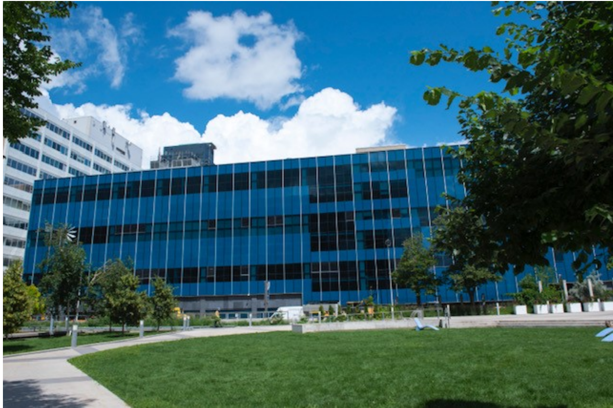
Police Headquarters Photo Credit: Winnipeg Police Service
