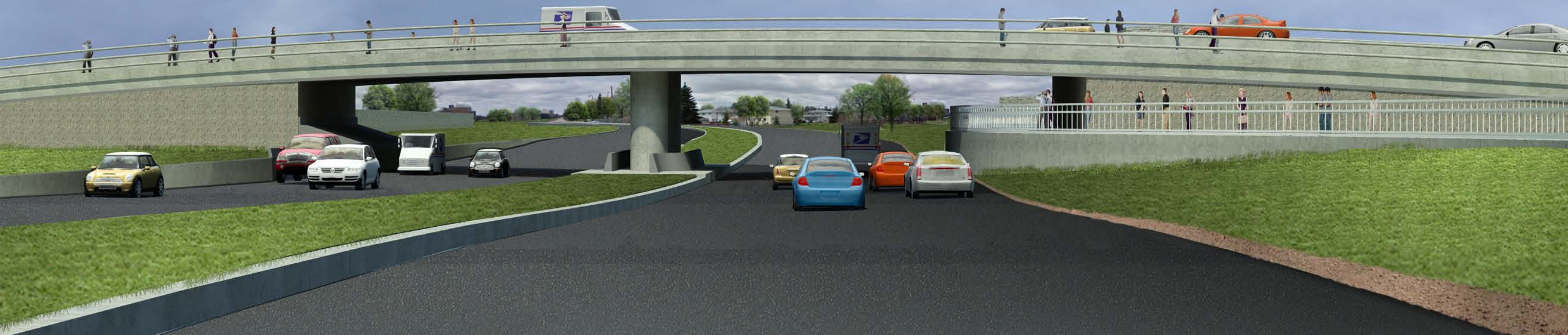
ROTHESAY BRIDGE - LOOKING WEST
